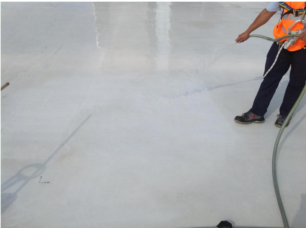
The cleaning with water only brought the surface at a good level, while the cleaning with the rag and water restored the surface to the original level, not possible without the application of the system PURETi Basecoat PURETi Clean, as evidenced by the following image.
