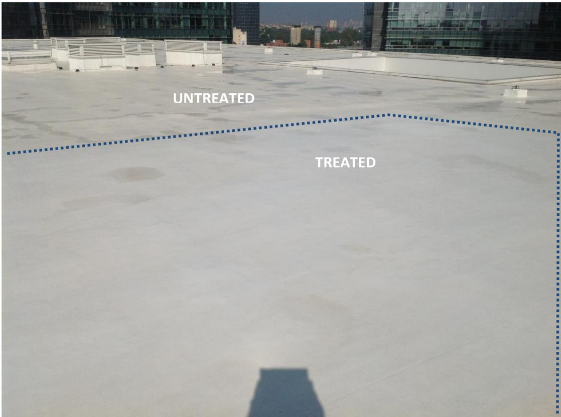
The surfaces treated with the photocatalytic system PURETi Basecoat \ PURETi Clean, appear much more clean and clear compared to untreated areas after 4 months from the application. The spots present are caused by puddles of water, because at night it rained
