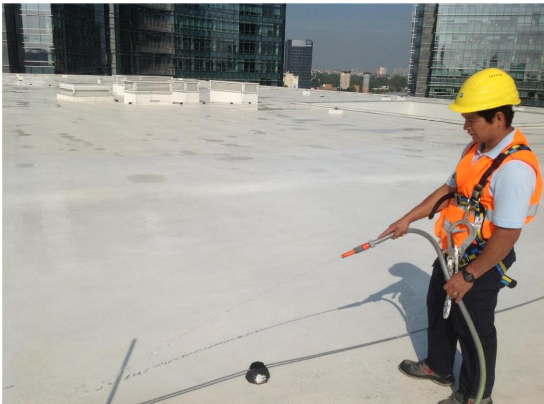
Later we proceeded to wash with water only the surface, as shown in the figure, then with a rag.
